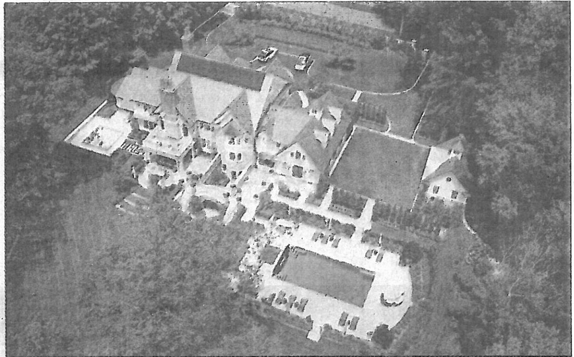
Hobbs, Inc., located on Grove Street, was awarded Fairfield County Project of the Year, for its work on the 10,000-square-foot luxury home pictured above. The awards are given out annually by the Home Builders Association of Connecticut. At right, the archstone bridge overlooks the cobblestone courtyard.
